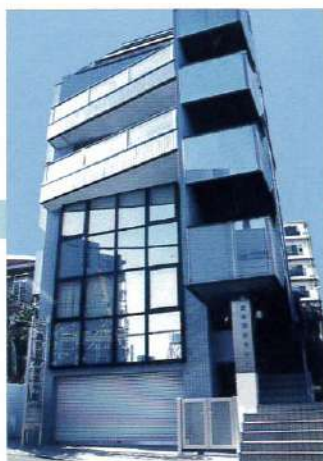
▲本校舎 Main Building
